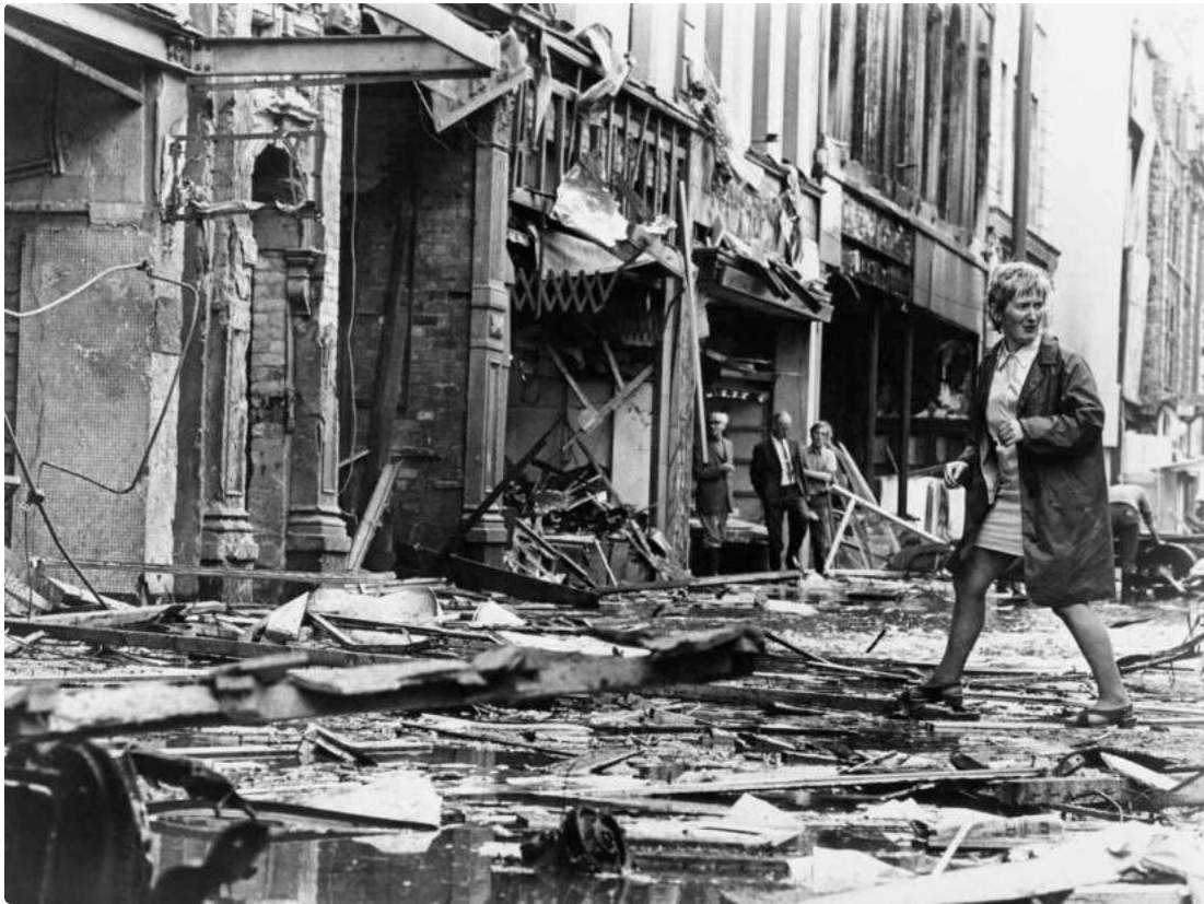
19. A woman anxiously treads through the rubble in the centre of Belfast, Northern Ireland, on 21 July 1972 following an IRA bomb attack. That day the IRA detonated no fewer than twenty-two bombs in the city, killing nine people and injuring a further 130.
